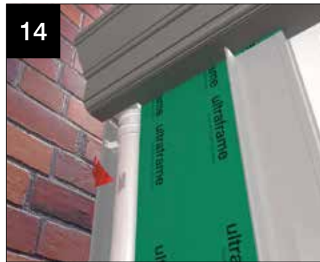
14 Fit concealed rainwater downpipe (if ordered)
