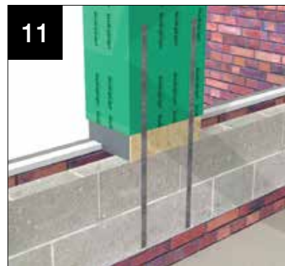
11 INLINE Fasten straps down inside of wall of inline column. Use suitable fixing.
