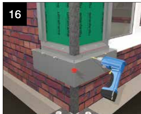
16 Fit plinths (picture shows trench not yet back filled)
