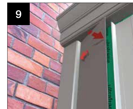
9 Push powder coated infill panel into abutment cladding and rock back against face of cladding clip.
