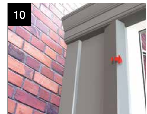
10 Clip on abutment cladding by locating inside clip first and rocking round the external clip as shown.
